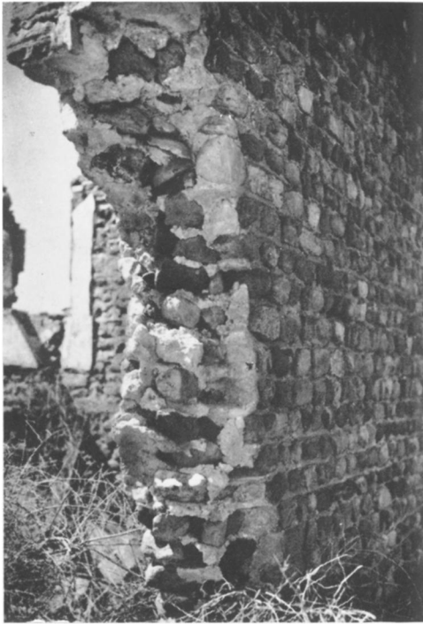
FIG. 1. Cobblestone masonry. (Author)
